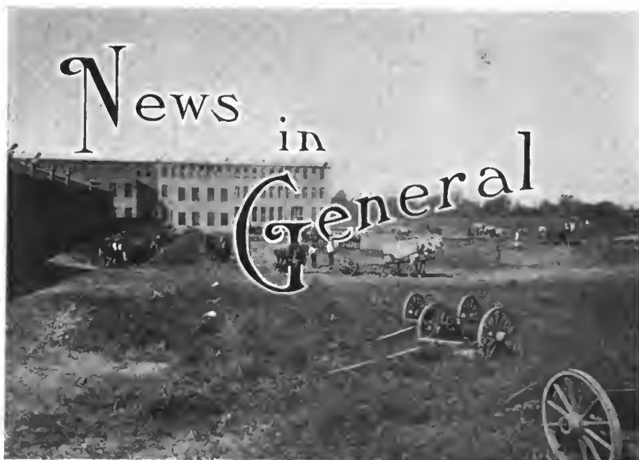
Breaking Ground for Addition to Overland Plant at Toledo, O.
